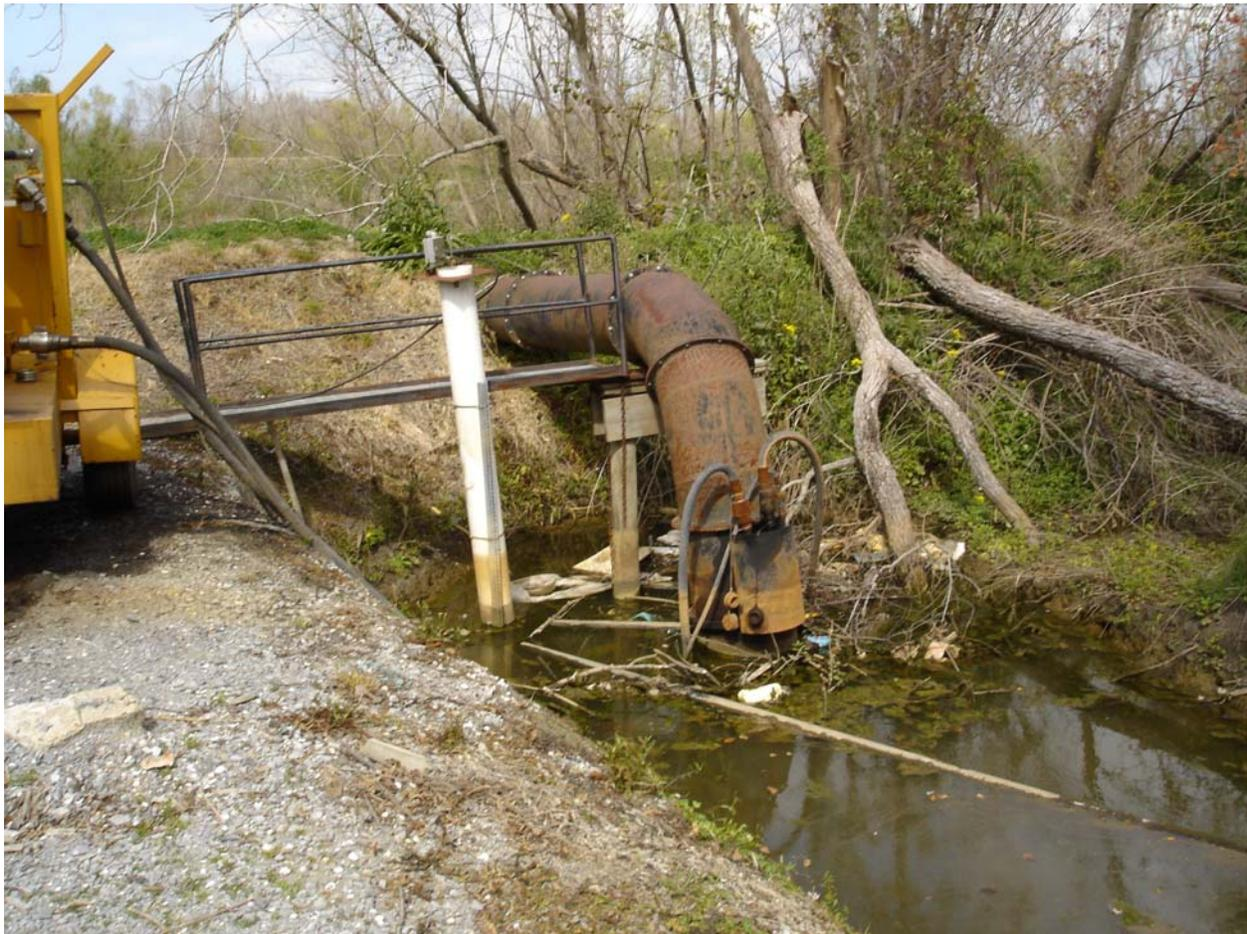
Figure 25. Hydraulically driven submersible pump.
