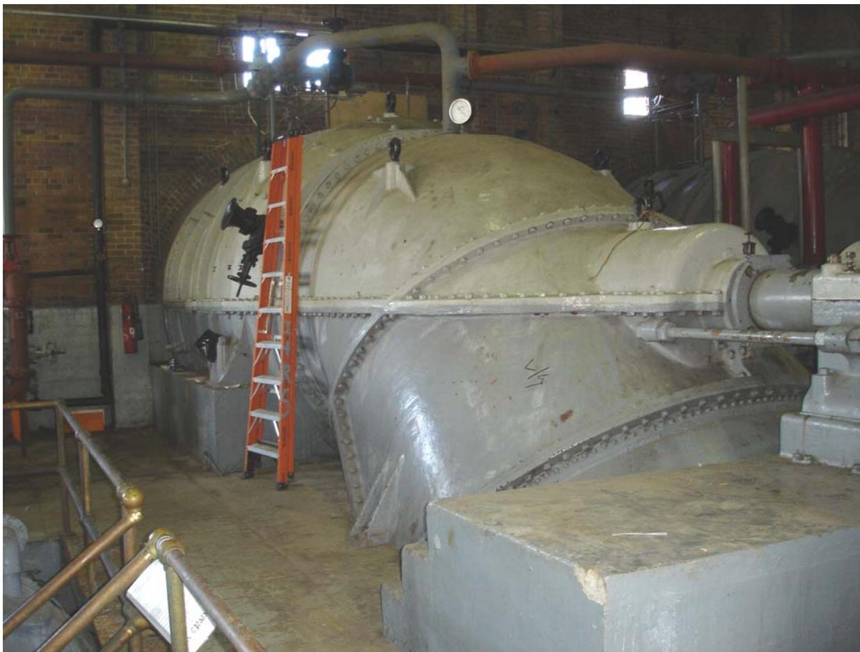
Figure 7. Large horizontal shaft pump.
